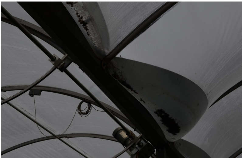
Figure 4. Condensation between the two layers will lead to water accumulation and eventually damage to the poly.
