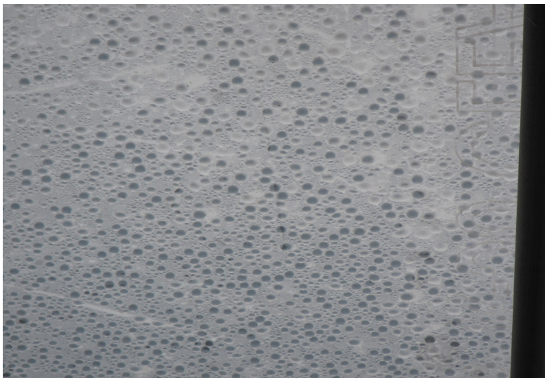
Figure 3. When inside air is used to fill the airspace between double-poly, condensation begins to form.
