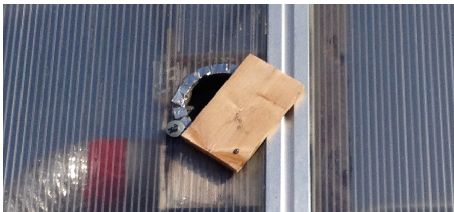
Figure 2. An example of a baffle on the outside air inlet for the inflation fan, this particular baffle is homemade, simply a piece of wood large enough to cover the entire hole and attached with a single screw at one corner. The baffle can be rotated to open or close the hole at any degree.
